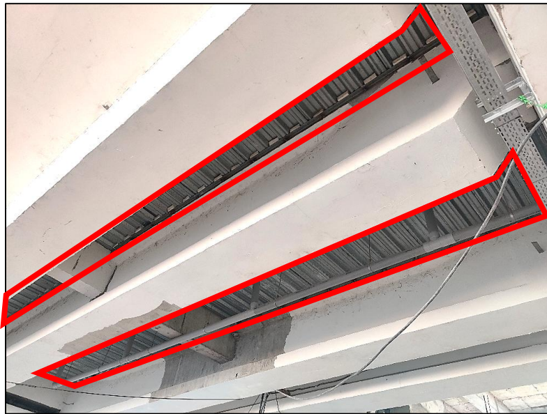
Figure 4: Stainless Steel Sacrificial Formwork (Source: By Author)
